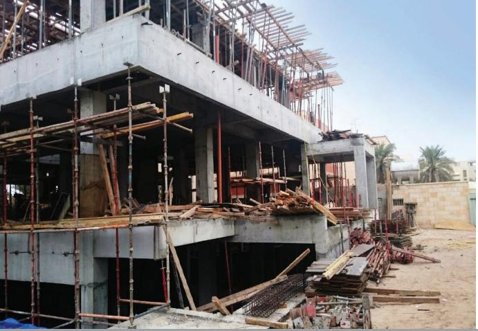
A residential villa in Shamiya district, built on 1000 m², consists of Basement, Ground floor, First floor, second floor and roof with swimming pool, the project is under construction.
